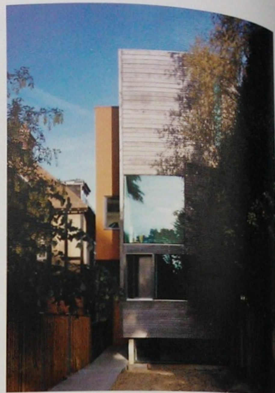
Terry Pawson Architects The Tall House, London, England, UK
